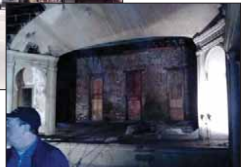
Below: Upstairs facing the stage. There is a full horseshoe balcony and the Opera House originally held an audience of 500.
